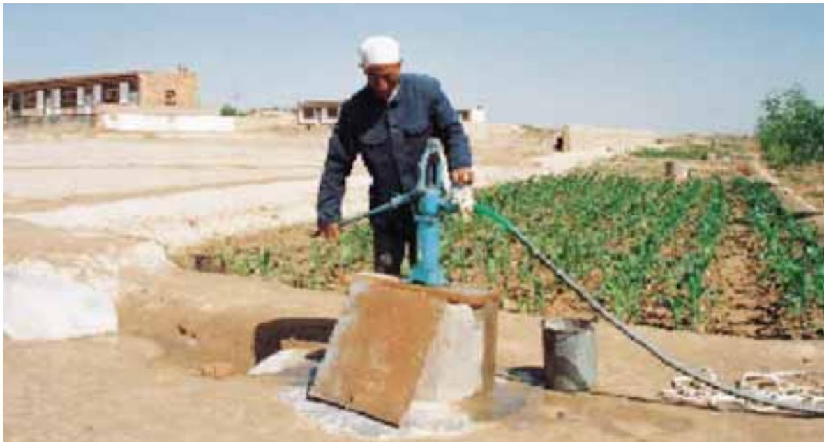
Figure 11: Manual pumping of water from a cellar
